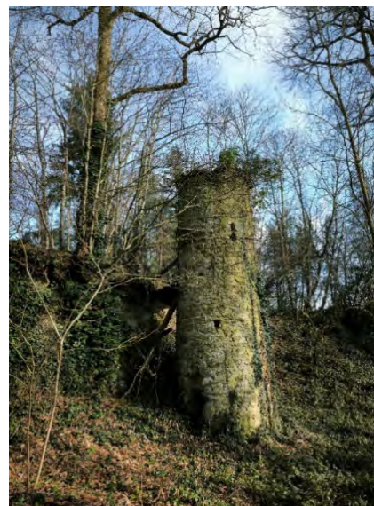
Station de pompage
